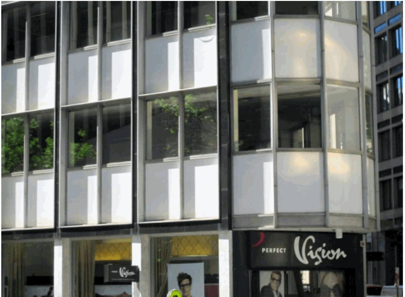
**Caption:** Detail of curtain wall cladding on west elevation and turning the corner
